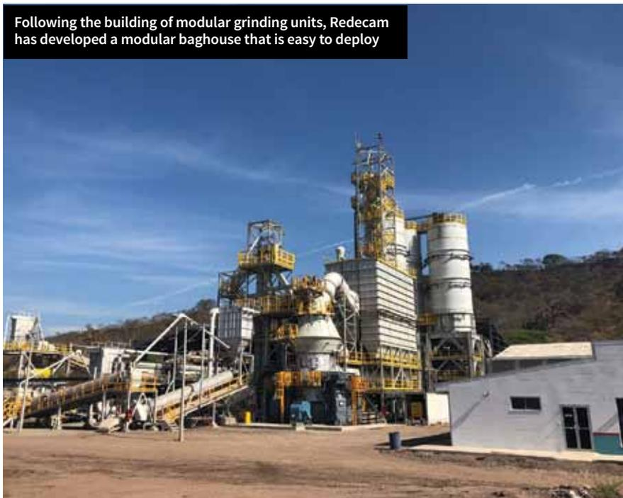
using only 7m bags, with the baghouse pre-assembled and shipped using only 15 standard 40ft containers.
